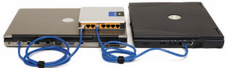
• Figure 22.10 A switch connected by UTP cable to two PCs
