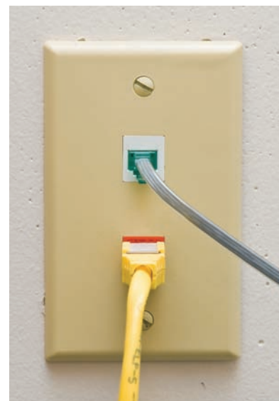
• Figure 22.30 Typical work area outlet
