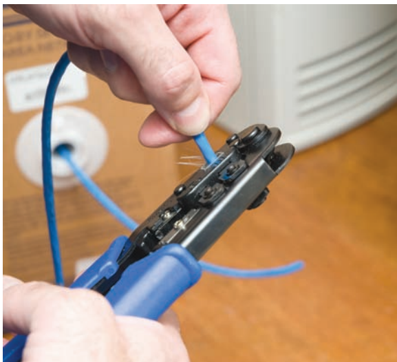
• Figure 22.26 Crimping the cable
